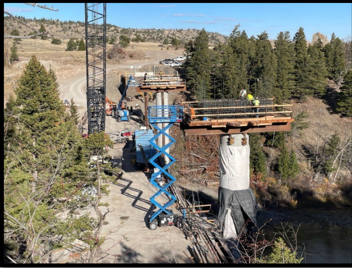
Piers 2 & 3 Caps Preparing for Concrete Placement
