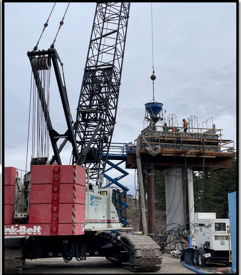
Pier 3 Cap Concrete Placement
