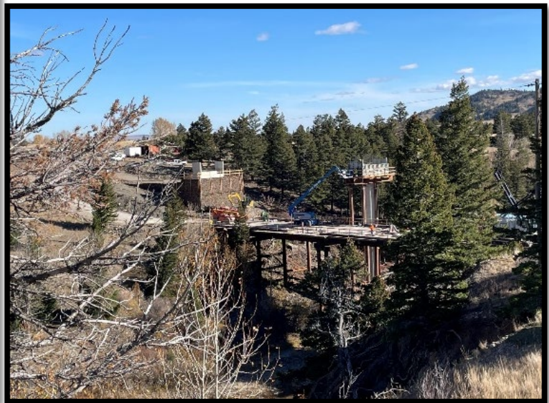
Pier 3 Cap Construction
