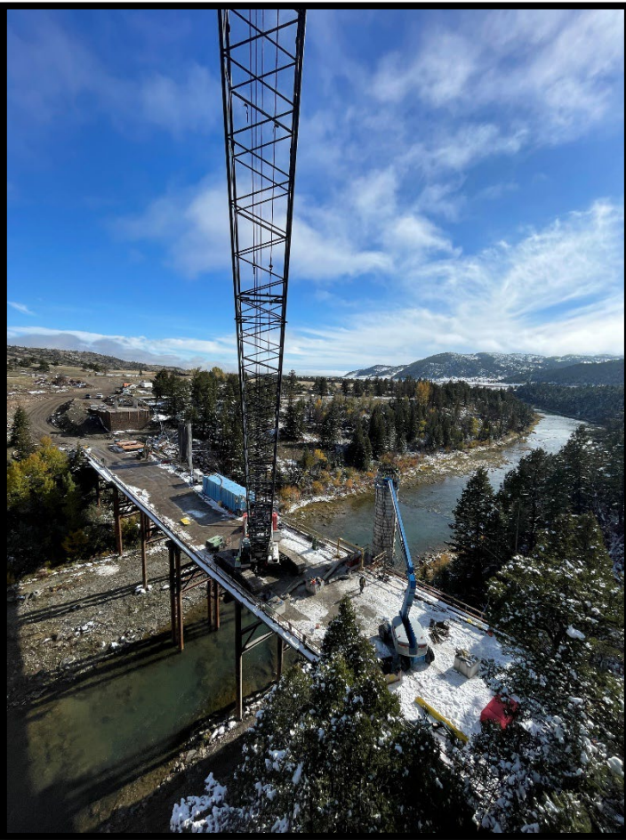
Ariel view of Recent Construction Activities
