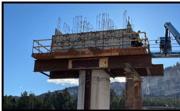
Pier 3 Cap Prepared for Concrete Placement
