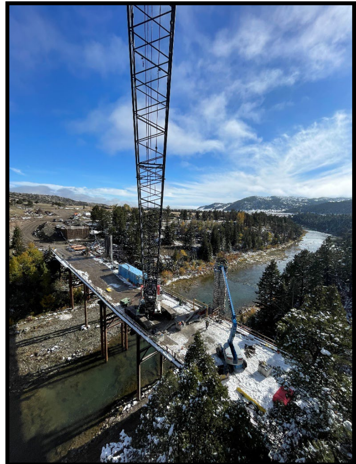
Aerial photo of current status of the project.
