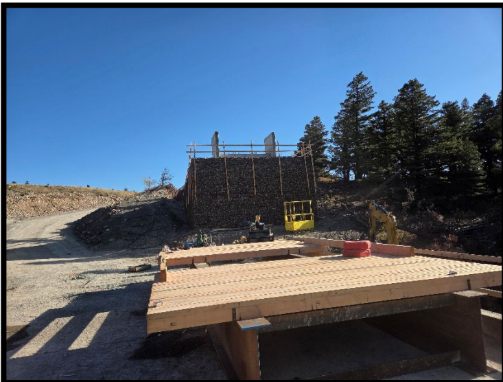
Pier Cap Falsework Deck Preparation
