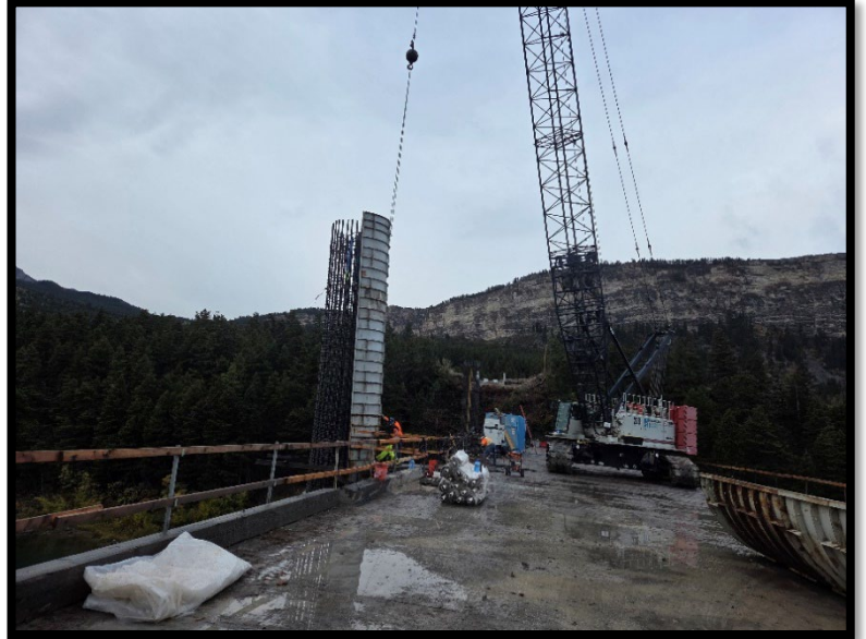
Repositioning of Pier 3 Column Forms
