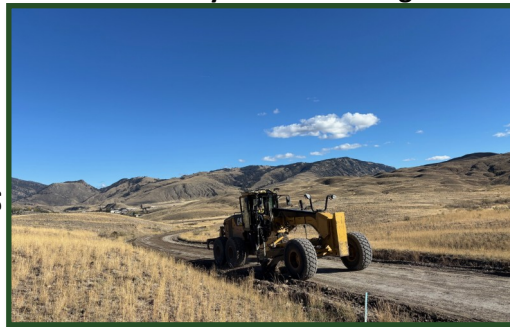
Surface Course Aggregate Compaction
