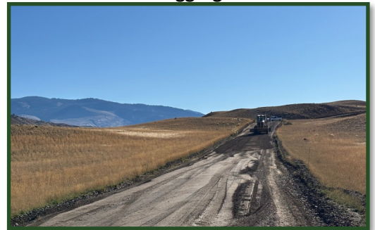
Surface Course Aggregate Compaction
