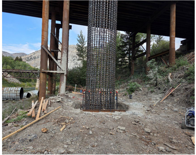
Pier 3 column cage being placed.
