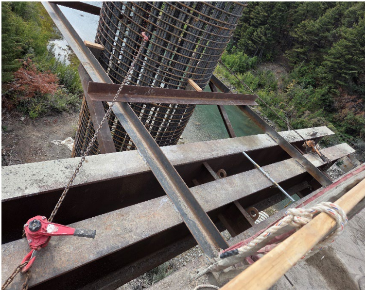
Pier 3 column cage placed and anchored off to the work bridge.
