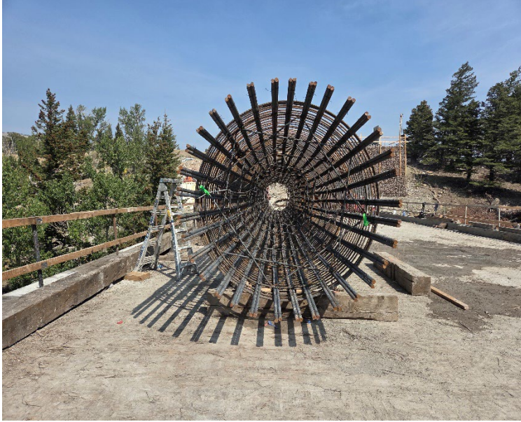
Column 3 reinforcing steel cage.
