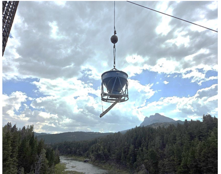
Concrete placement into upper portion Pier 3 drilled shaft .
