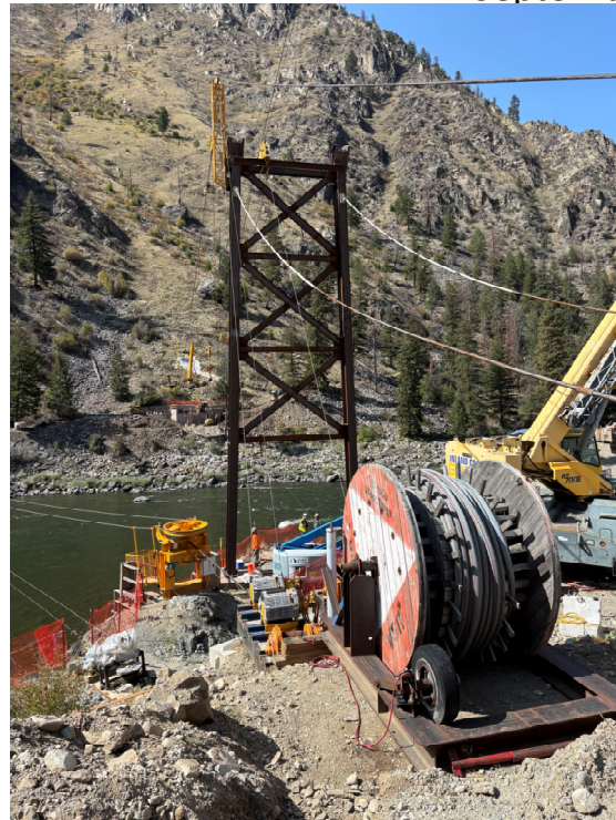
Getting the Temporary Works and the first Main Cable spool in place.
