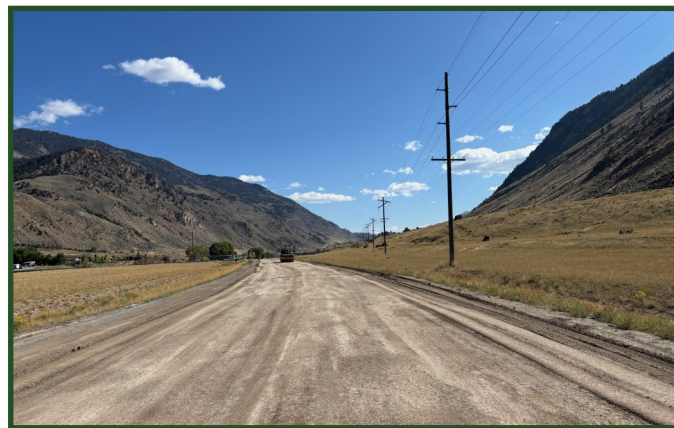
Surface Course Aggregate after Compaction
