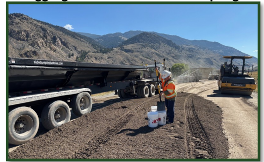
Surface Course Aggregate after Compaction
