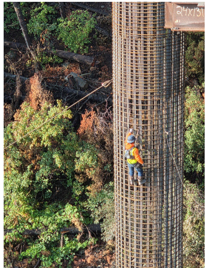
Worker on Pier 2 Column Cage Securing Guy Wires for Stability.
