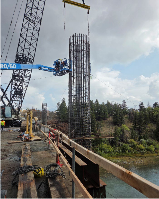
Installing Pier 2 Column Reinforcing Steel prior to Concrete Placement.
