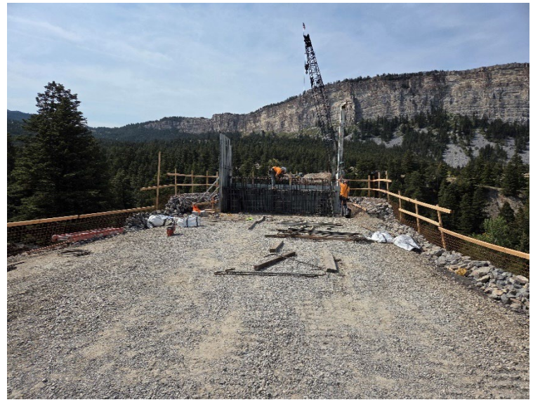
Abutment 4 (east side) Placement of Reinforcing Steel and Forms
