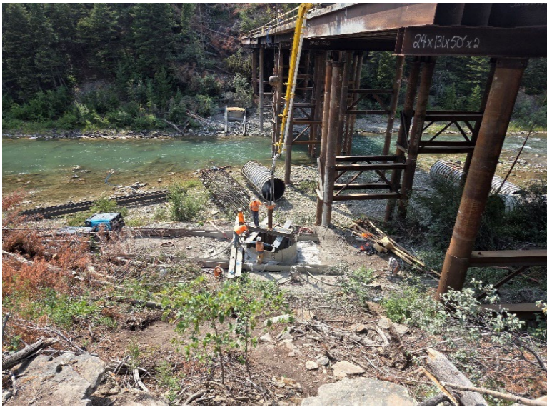
Concrete Placement in Drilled Shaft at Pier 3
