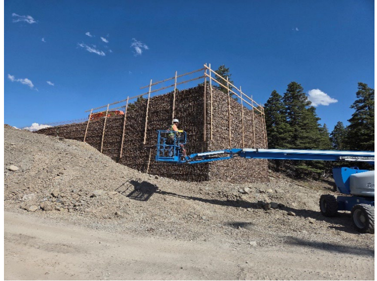
Abutment 4 MSE Wall (east side) Construction
