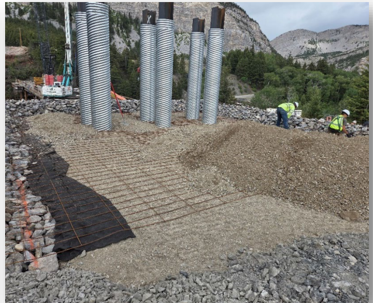
MSE wall construction on the east side at approximately 20% complete.
