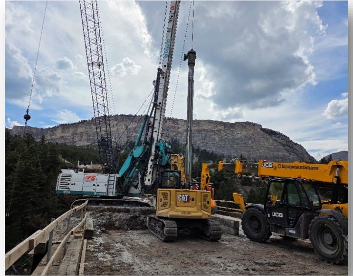
Drilling Pier #3 Drilled Shaft from the Temporary Work Bridge with significant support apparatus.
