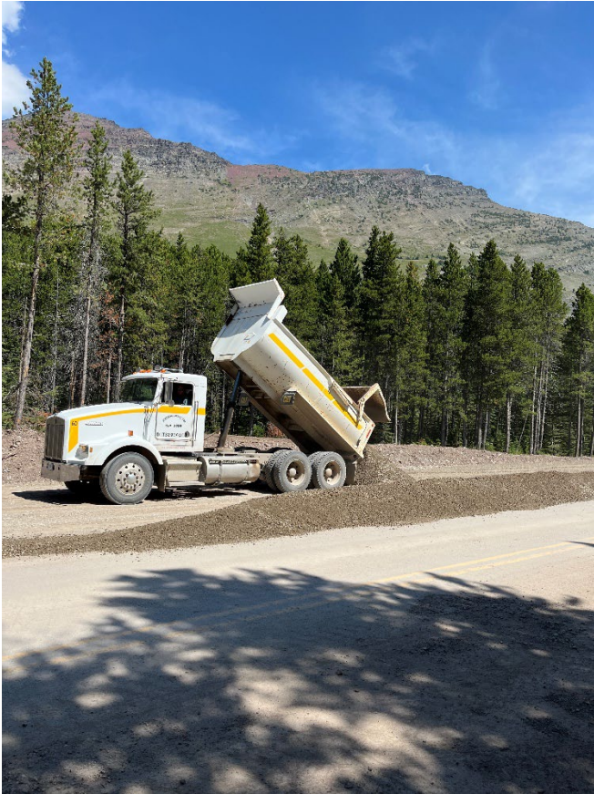
Spreading base material on new parking area
