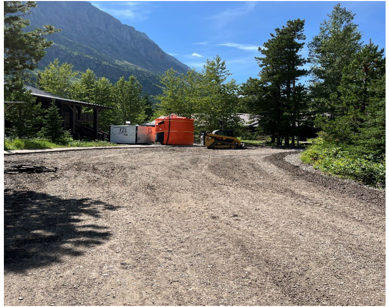
Grading pulverized asphalt in the Admin Loop
