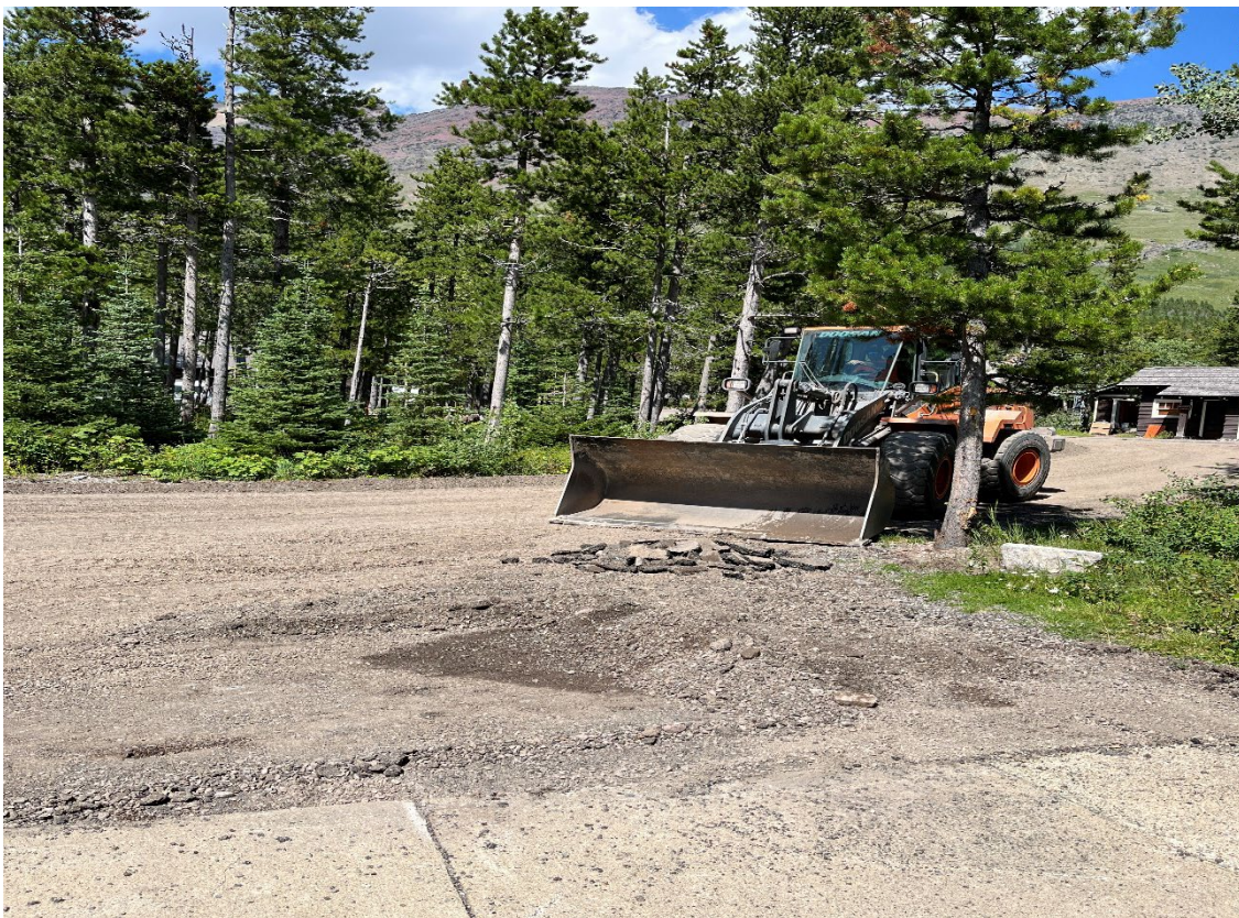
Grading pulverized asphalt in the Admin Loop
