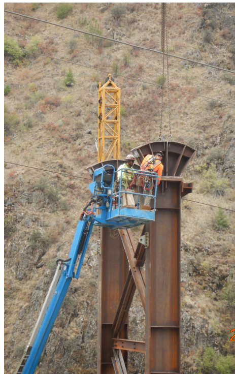
Setting the Tower Saddles and a Abutment 1 Saddle Bearing and Anchor Block Vault.
