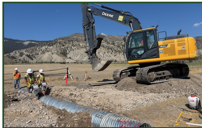
Culvert Installation
