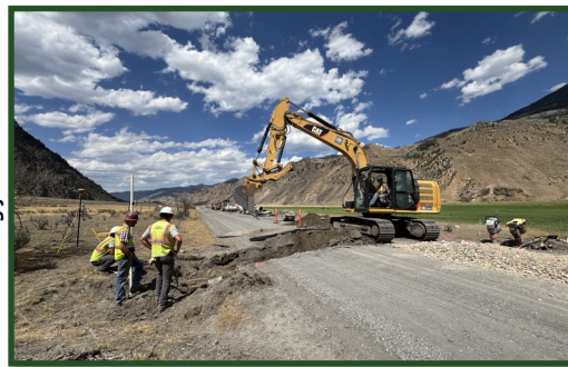
Existing Culvert Removal
