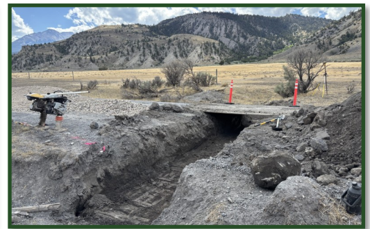
Existing Culvert Removal
