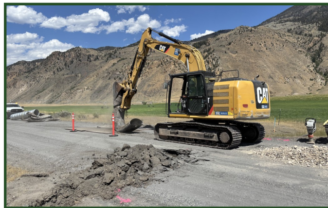
Existing Culvert Removal
