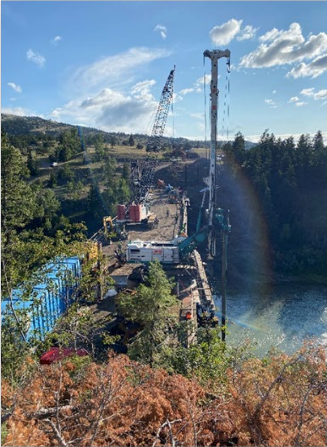
Drill Rig on Work Bridge 40' above Pier #2
