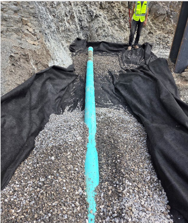
MSE Wall Underdrain Construction
