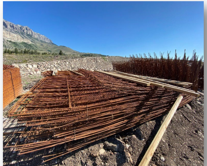
Components for Mechanically Stabilized Earth wall
