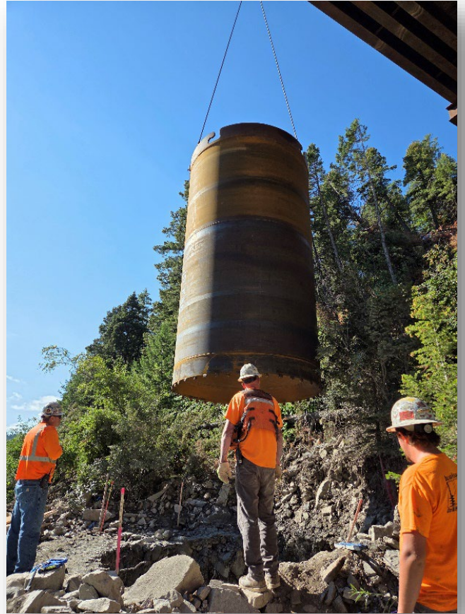
Lowering Steel Casing Down to Pier #2 Construction
