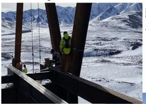
Checking the torque on the bolts at diagonal connection L1'
