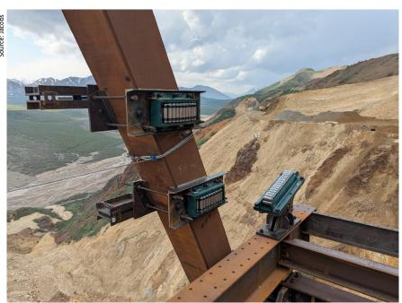
Lateral guide rollers attached to south L0-U1 and vertical rollers at L0.
