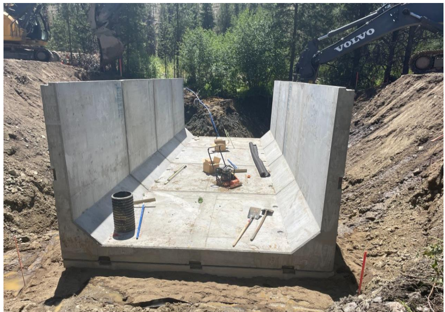
Boundary Box Culvert Installation
