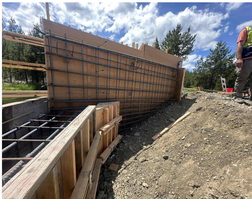
Concrete Formwork and Rebar
