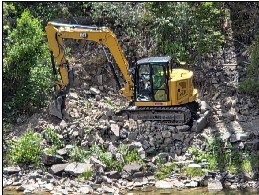
Clearing for Drilled Shaft at Pier #2 (west side).
