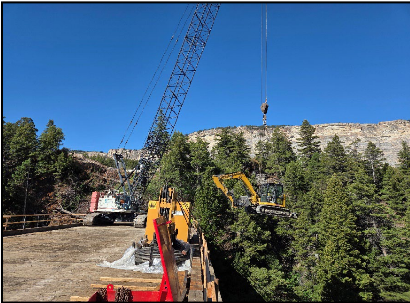
Lowering a small excavator to the work zone to minimize the impact to the environment.
