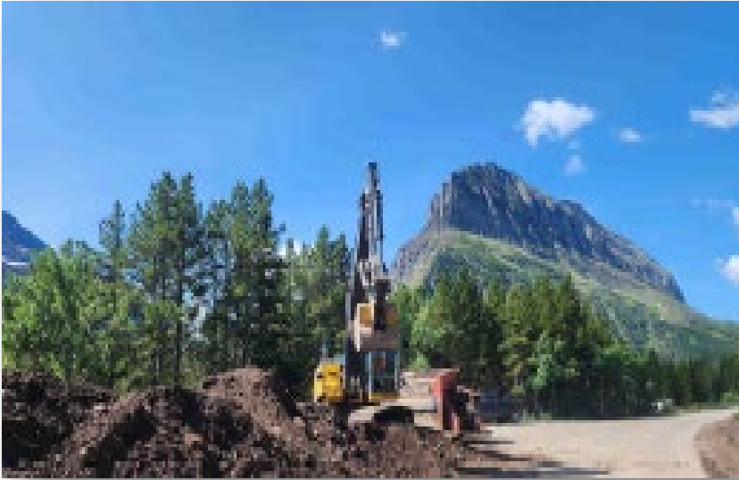
Screening Topsoil
