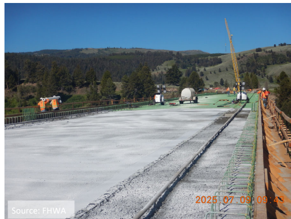
Application of Curing Compound.
