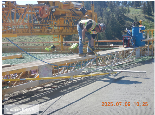
Applying Tined Finish.
