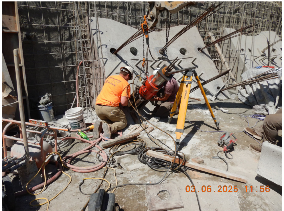
Setting up for Abutment 1 PGA proof test
