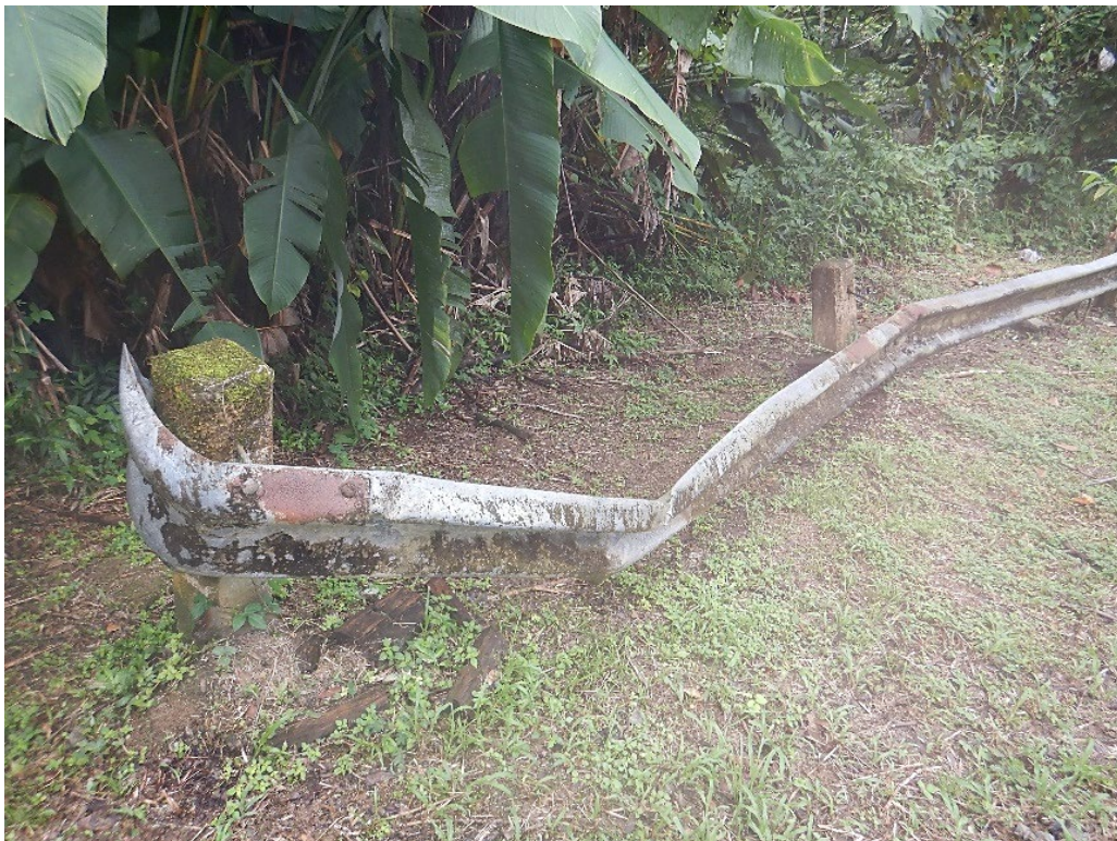
Figure 6. Example of damage to steel beams of the current guardrail system.
