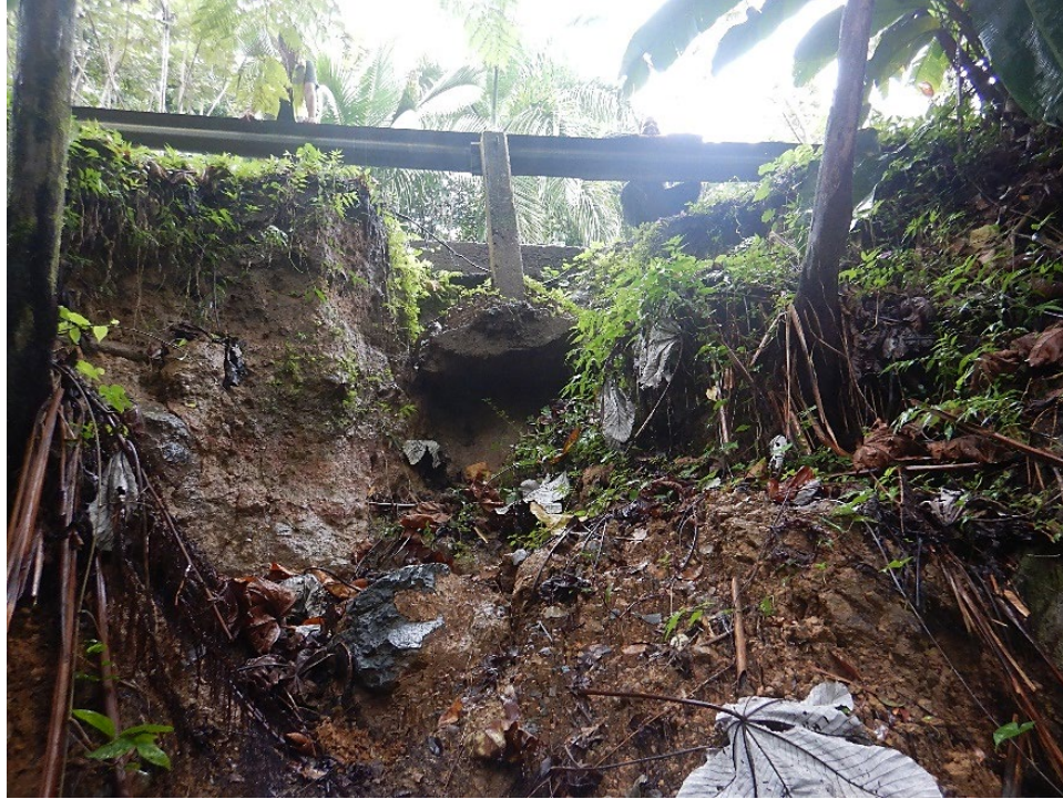
Figure 7. Guardrail damage caused by a landslide.
