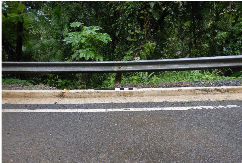
Figure 4. Example of new concrete curbs & gutter design.
