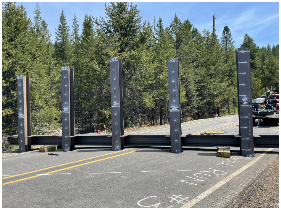
Driven Piles at Bull Rune #3
