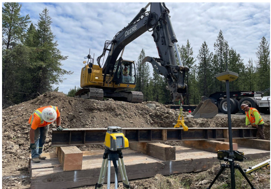
Bull Run #4 Temporary Bridge Footings
