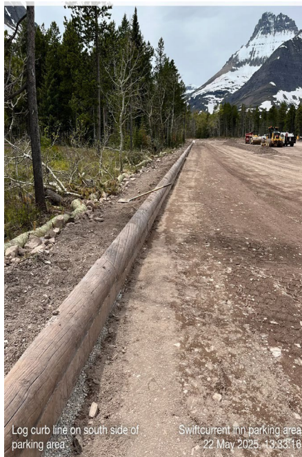
Pre-Cast Log Curb Placement at Swiftcurrent Inn Parking Area
