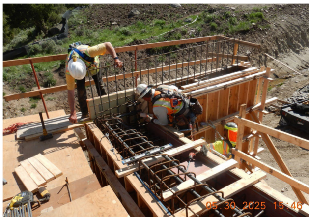
Rebar/Formwork inspection at Abutment 1 Backwall/Stubwalls
