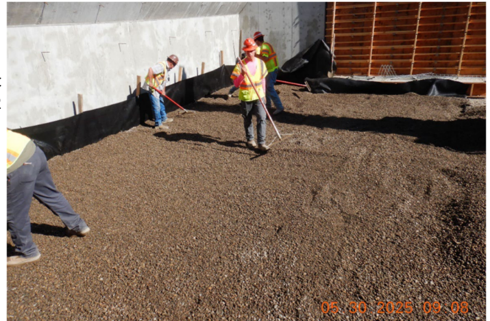
4th Layer of GRS backfill at Abutment 2
