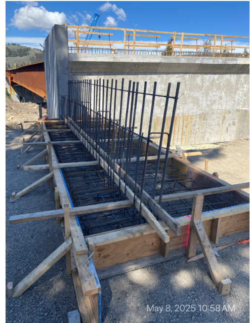
Abutment 2 wingwall footing formwork
