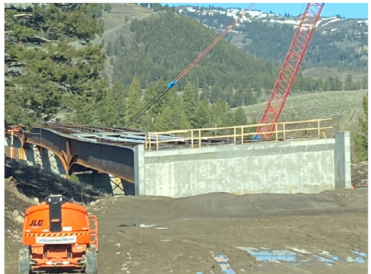
Placement of precast deck panels at Pier 2
