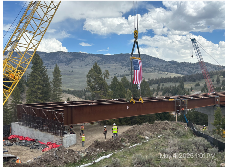
Placement of final girder at Abutment 1
