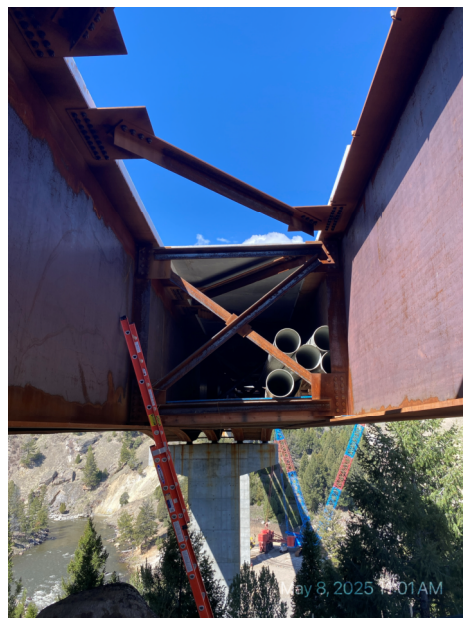
False decking in bay 4 with underdrain pipe ready to install.
