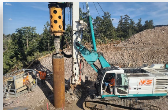
Drilling Shaft for Socketed Pile
