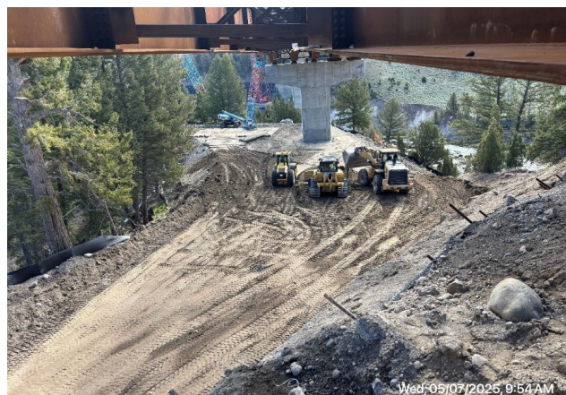
Backfilling the slope at Pier 1
