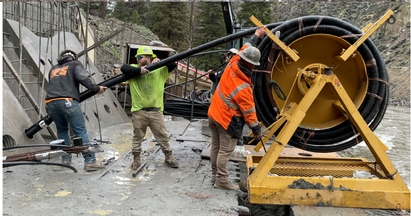
Installation of the tendons in the PGAs
