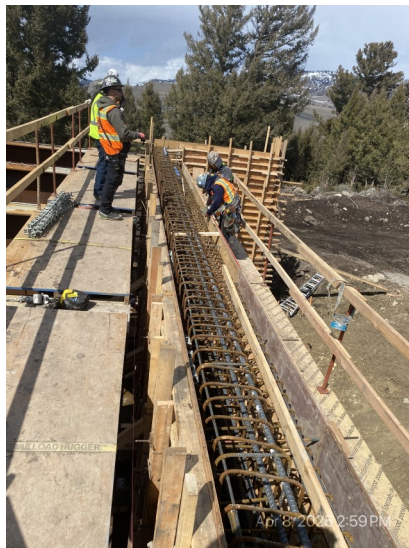
Final rebar and form inspection prior to concrete pour
