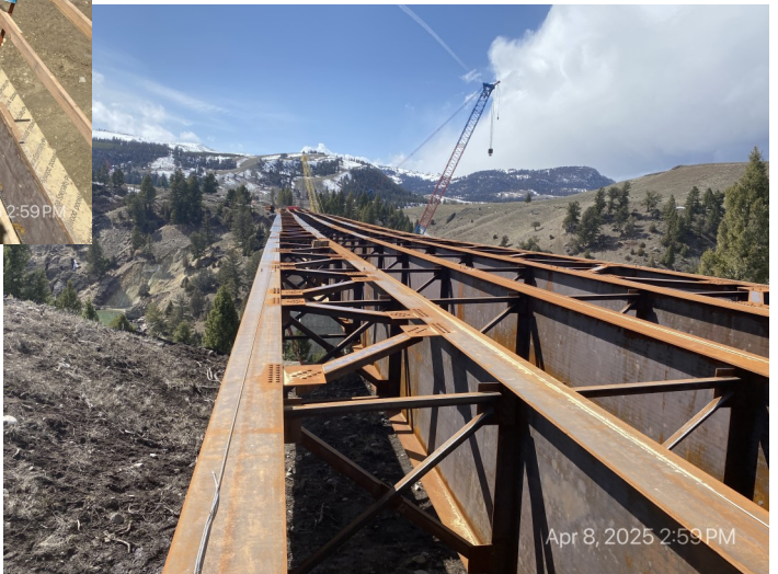
View of new girders from Abutment 2
