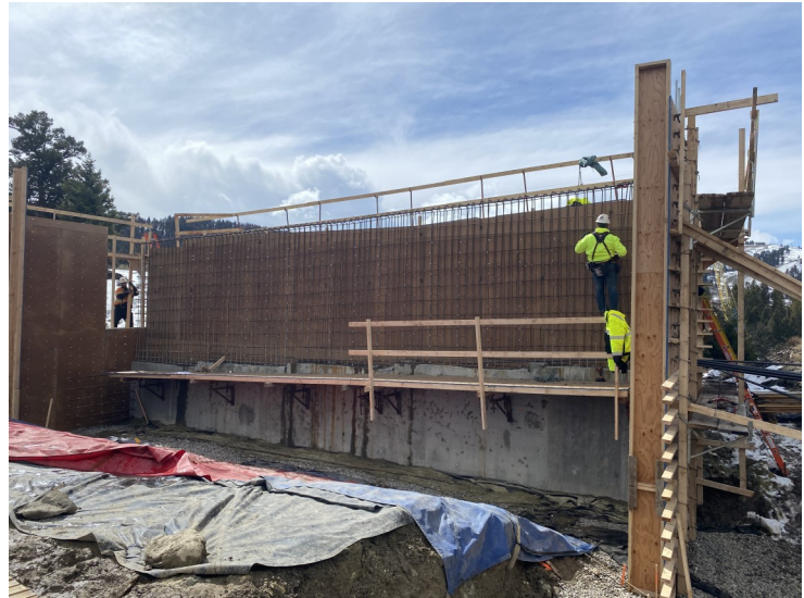
Formwork and rebar at Abutment 2 Back and side walls
