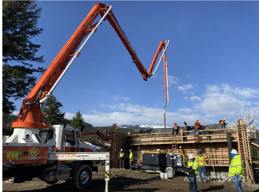
Daytime picture of concrete pour at abutment 2
