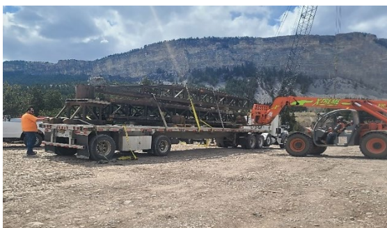
Pile driving hammer being unloaded
