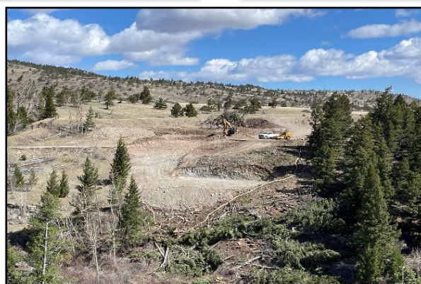
Excavation of Access Road for Temporary Bridge and Abutment 4
