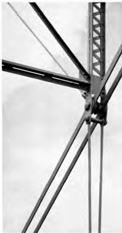
The Fort Keogh Bridge (Description 16) is an excellent example of the pin-connected Pennsylvania truss used frequently for long spans throughout Montana in the early 20th Century. (Photograph Jet Lowe).
