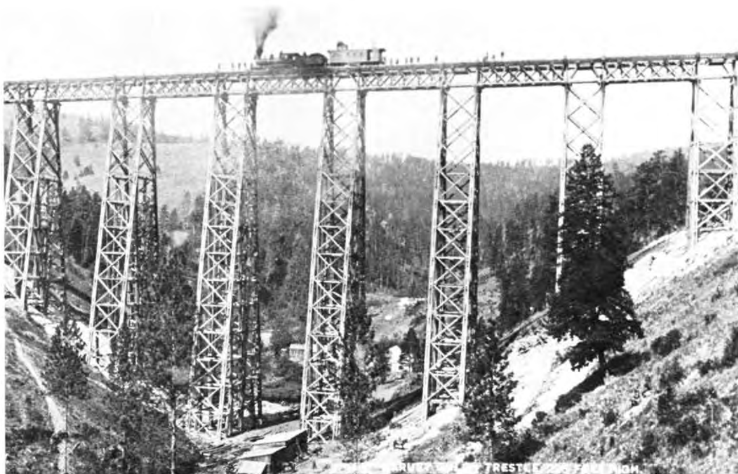
The 1883 wooden trestle at Marent Gulch near Missoula was the most spectacular structure of the new Northern Pacific transcontinental line across Montana. (Minnesota State Historical Society Archives).
