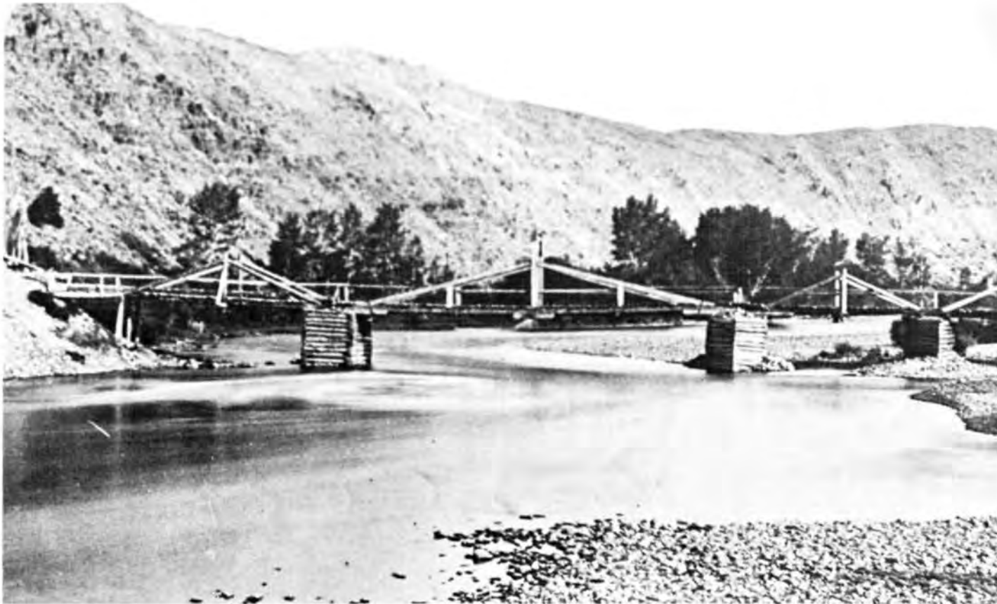
Browne's Bridge (Description 1) over the Big Hole River was an important part of the network of southwest Montana roads connecting the gold fields with Corrine, Utah and with Fort Benton on the Missouri River. The king post spans survived until 1921. (Montana State Historical Society).
