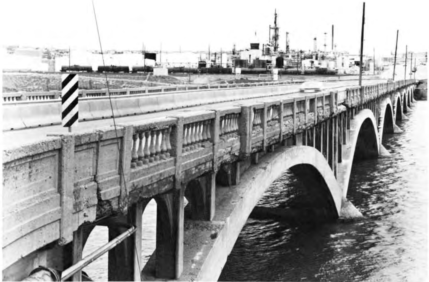
The Tenth Street Bridge (Description 11) over the Missouri River in Great Falls is the longest surviving multi-span, open spandrel concrete arch bridge in Montana. It and the recently demolished First Avenue North Bridge were built in 1920. (Photograph Jet Lowe).
