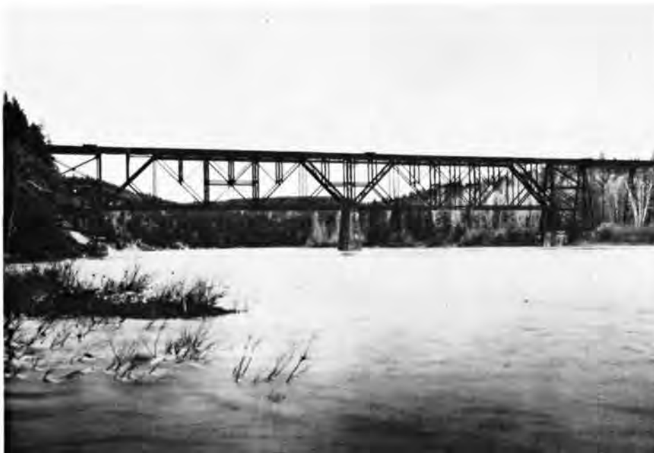
This Baltimore deck truss bridge across the Flathead River at Coram was built by the Great Northern Railroad in 1898. (Photograph Jet Lowe)
