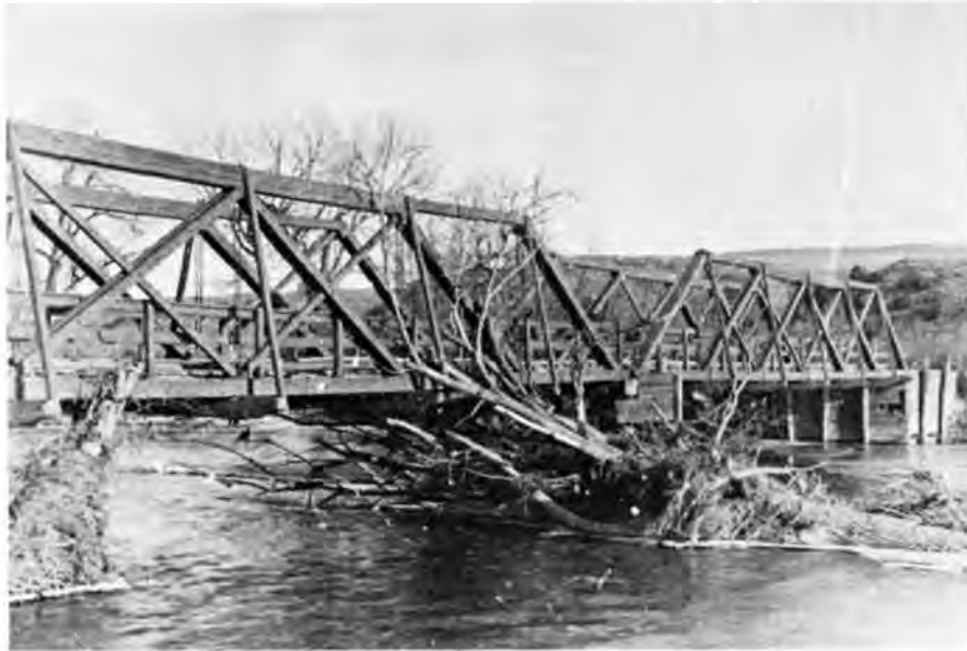
This wooden Howe pony truss over the lower Clark's Fork of the Yellowstone Carbon County line is typical of the Howe pony trusses built in 19th Century Montana. (Montana State Historical Society).
