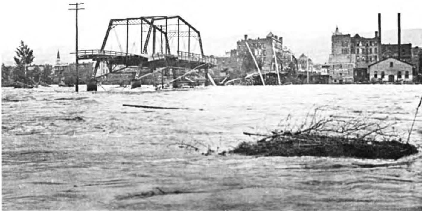
The Higgins Avenue Bridge in Missoula, built by O. E. Peppard in 1890's was washed out in the Flood of 1908. Two of the spans were salvaged and moved upstream to Van Buren Street (Description 53) where they stand today. (Stereoscopic photographs in possession of Ray Calkins, President, Butte Historical Society).
