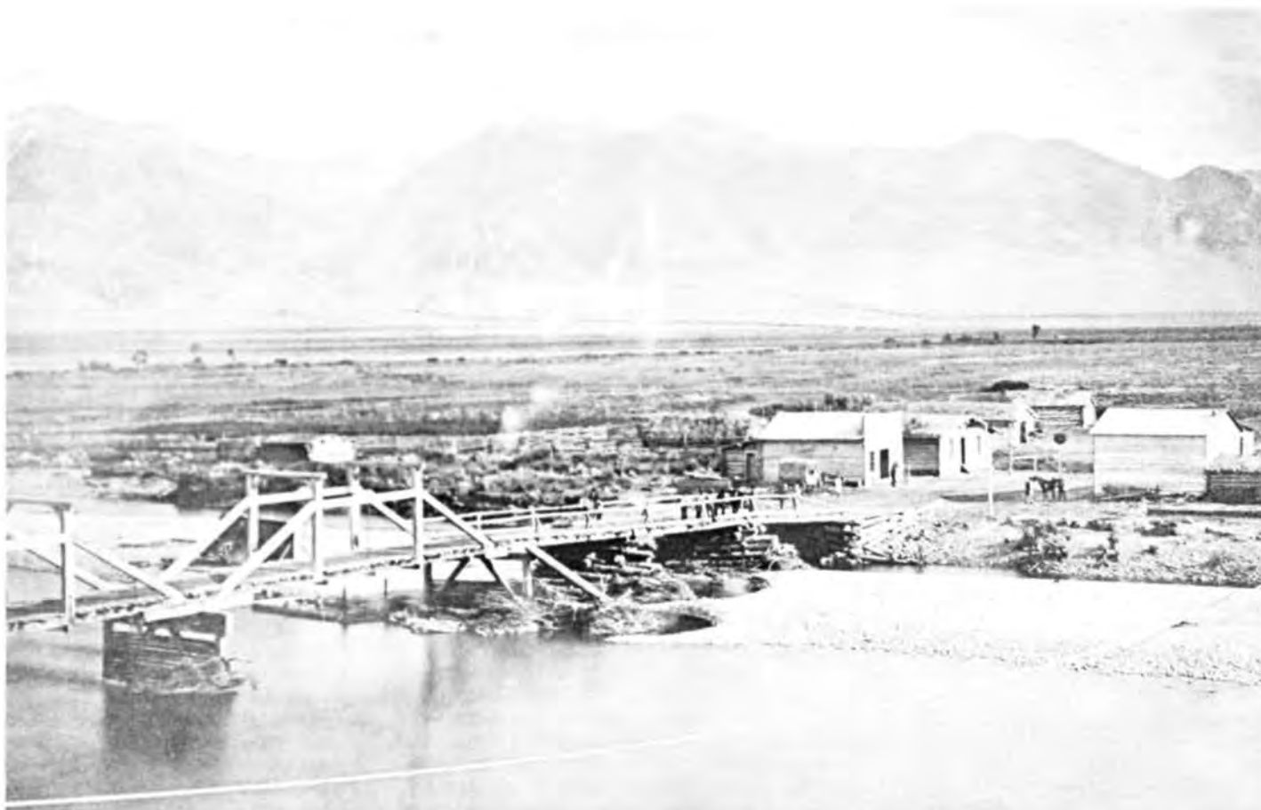
Parson's Bridge over the Jefferson River was, in 1866, a prominent southwest Montana landmark during early settlement. It is typical of the bridges built by local bridge builders. Note that the middle floor beam is supported by a tensile member suspended from the upper chord which acts as a beam. (Montana State Historical Society).
