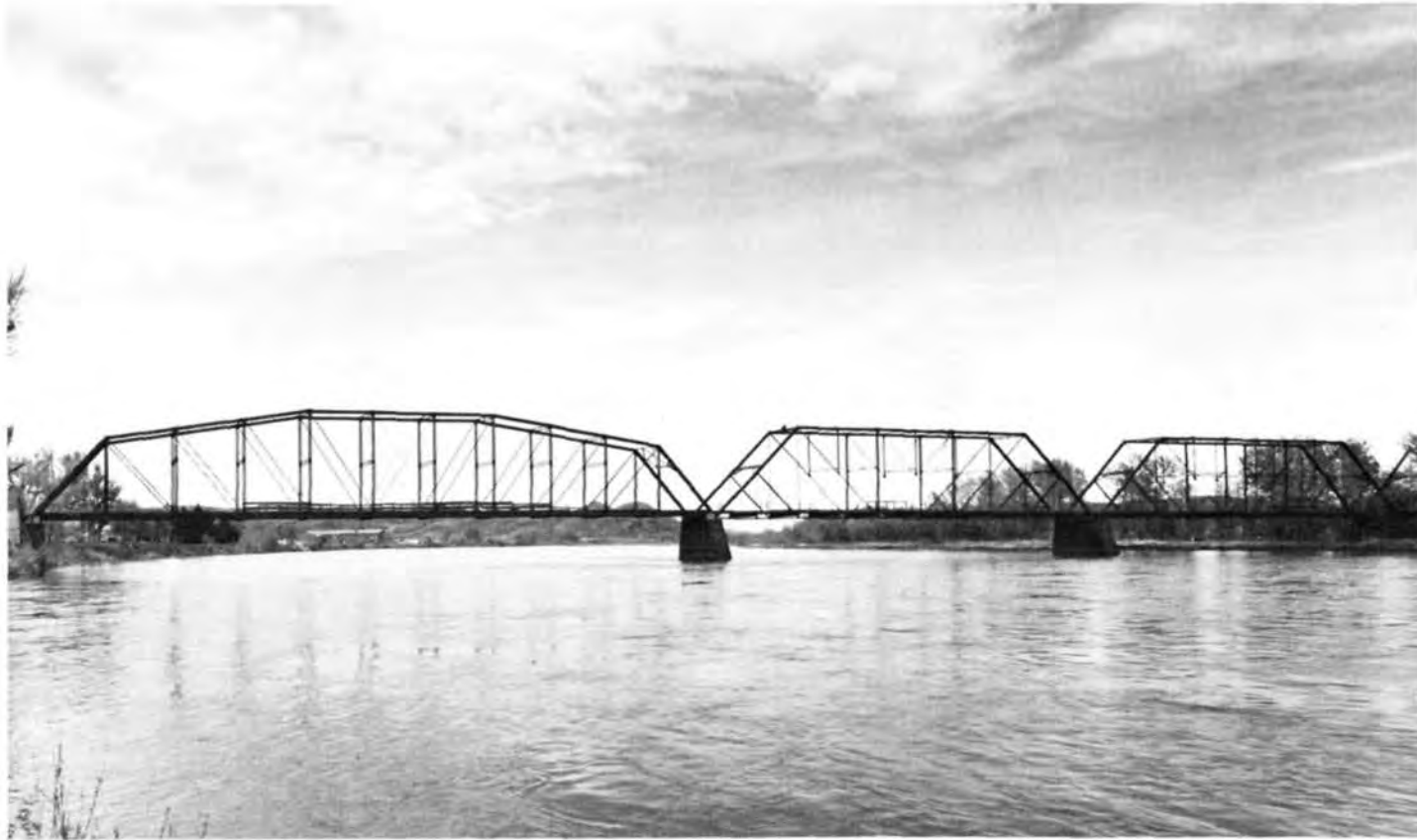
The Fort Benton Bridge (Description 14) was built in 1888 by the Milwaukee Bridge and Iron Company. The Parker span on the left was built in 1925. The Baltimore spans on the right are original to the structure. (Photograph Jet Lowe).
