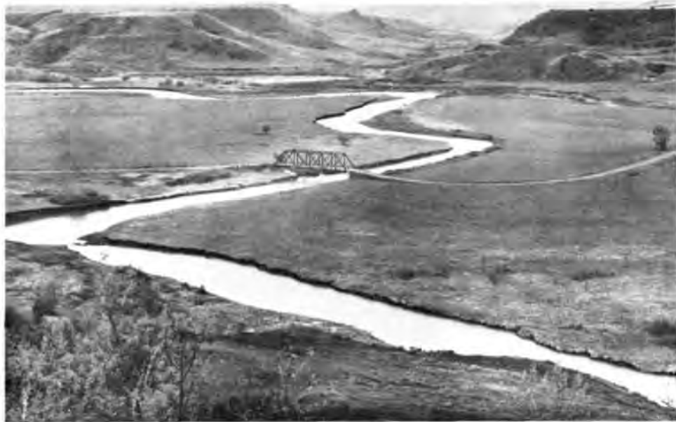
The boom in bridge building that accompanied the county splitting of the Homestead Era left many steel truss bridges in remote places such as the Deerfield Bridge over the Judith River. (Photograph Jet Lowe).
