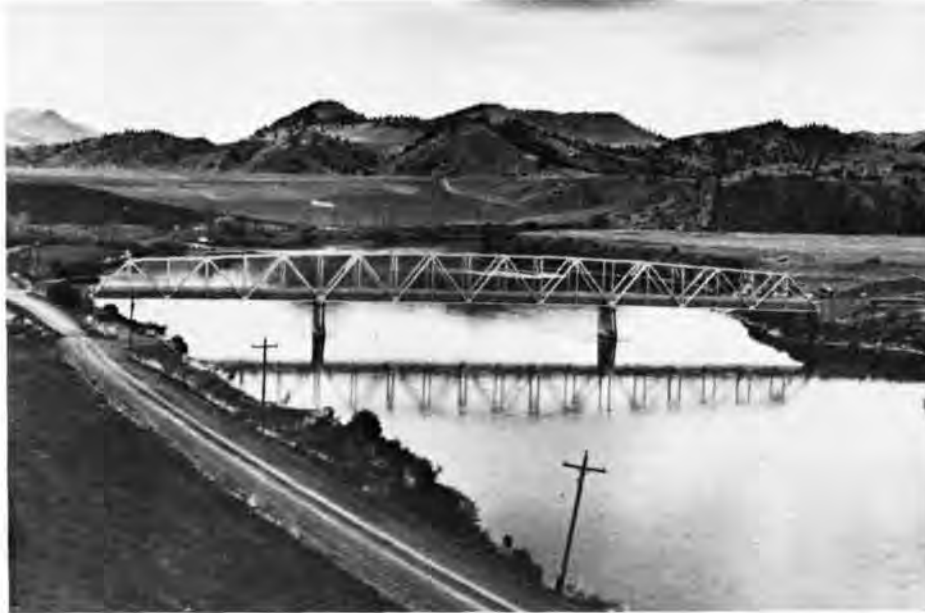
The Wolf Creek Bridge (Description 39) over the Missouri River was built in 1933. It was the first multi-span, continuous truss bridge built in Montana. (Photograph Jet Lowe).
