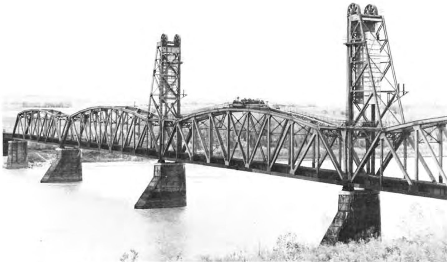
The Fairview Bridge in North Dakota crosses the Yellowstone River just over the Montana/North Dakota border. It is similar to, but smaller than, the Snowden Bridge (Description 65). The Fairview Bridge was also designed by Waddell. (Photograph Jet Lowe).
