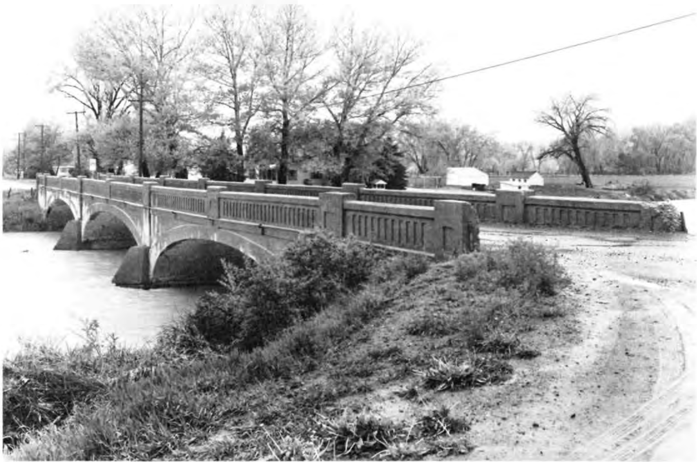
The Fromberg Bridge (Description 9) was built in 1914, very early for reinforced concrete arch construction in Montana. (Photograph Jet Lowe).
