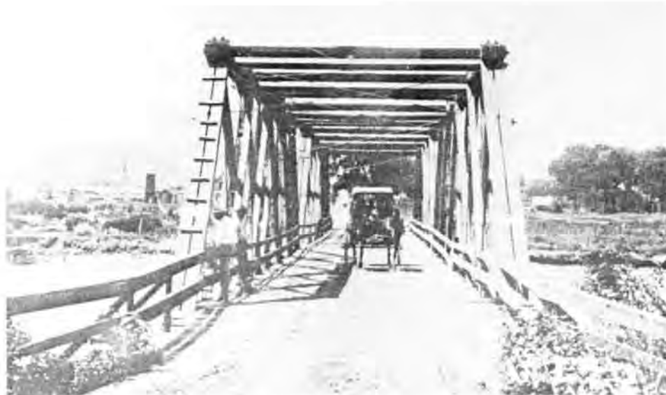
This wooden Howe through truss at Fromberg was replaced by the present concrete arch bridge (Description 9). The Howe truss is typical of 19th Century Montana wooden Howe through trusses, (Fromberg Service Club).
