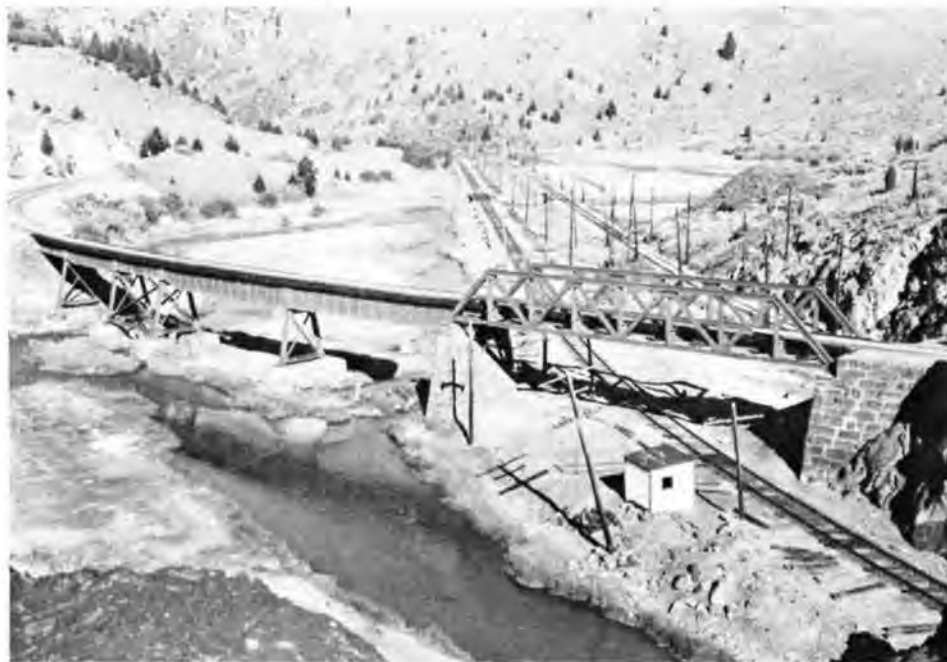
The Butte, Anaconda and Pacific Railroad Bridge (Description 70) over Silver Bow Creek and the Burlington Northern Railroad was built in 1897. It is the only truss bridge owned by the B.A. & P. (Photograph Fred Quivik).
