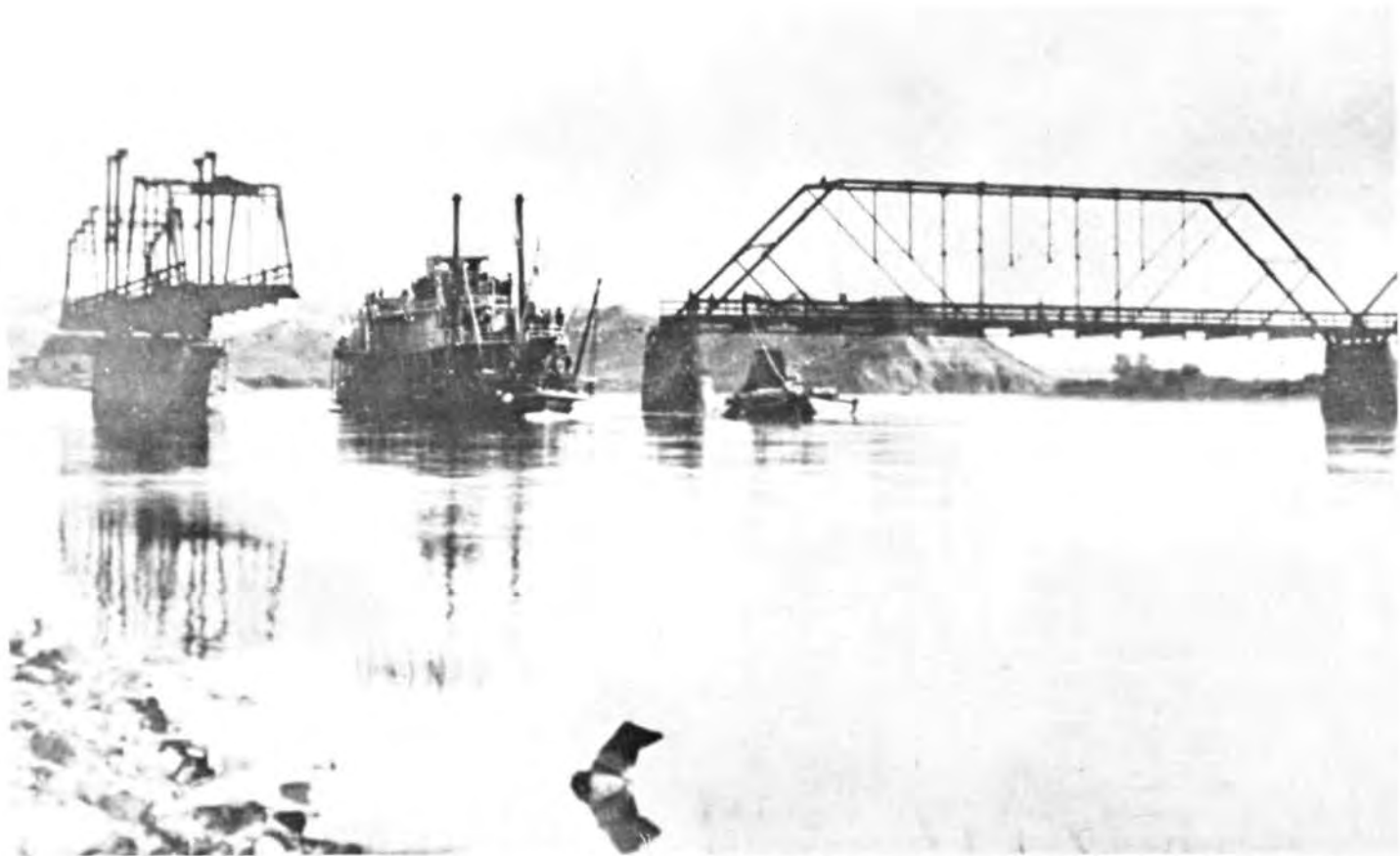
The swing span of the 1888 Fort Benton Bridge (Description 14) did not open to allow a river boat to pass until 1908. (John Lepley, Fort Benton Historical Society).
