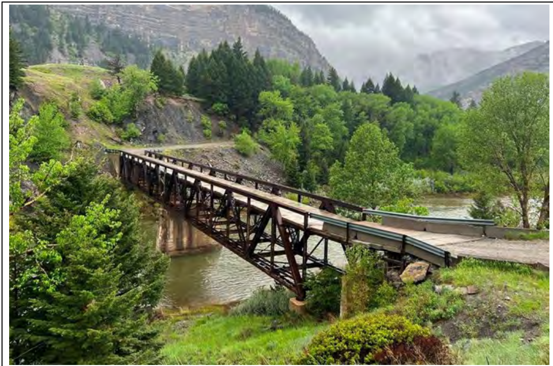
Figure 6. Sun River Bridge (24TT199), southeast face; view west. Photo by Jeannie Larmon, 5/25/2023.
