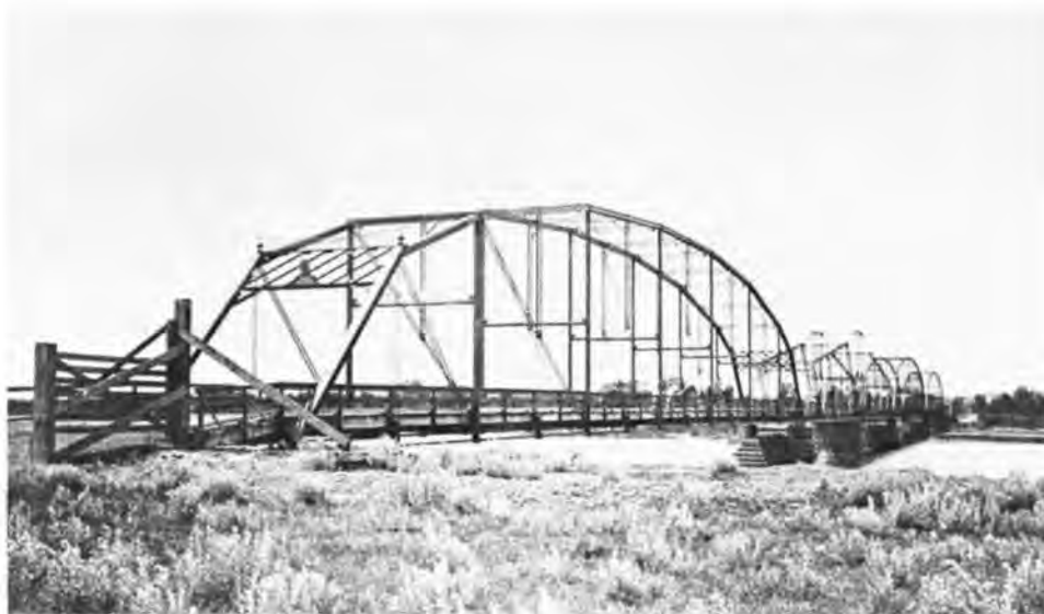
The 1895 Yellowstone River Bridge at Glendive (Description 20) was built by the King Bridge Company of Cleveland Ohio and included a swing span. (Montana State Historical Society).
