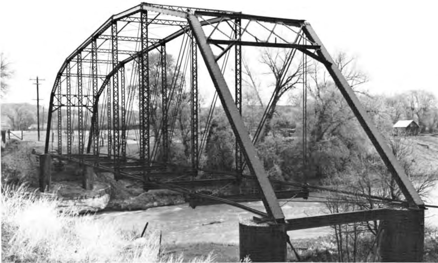
Originally, Sample's Crossing was merely a ford of the Judith River. The first bridge at the site was built in 1890 in direct response to the construction of the Fort Benton Bridge (Description 14). This pin-connected Parker through truss bridge (Description 22) was built in 1899 by the King Bridge Company. It was abandoned in 1948. (Photograph Jet Lowe).
