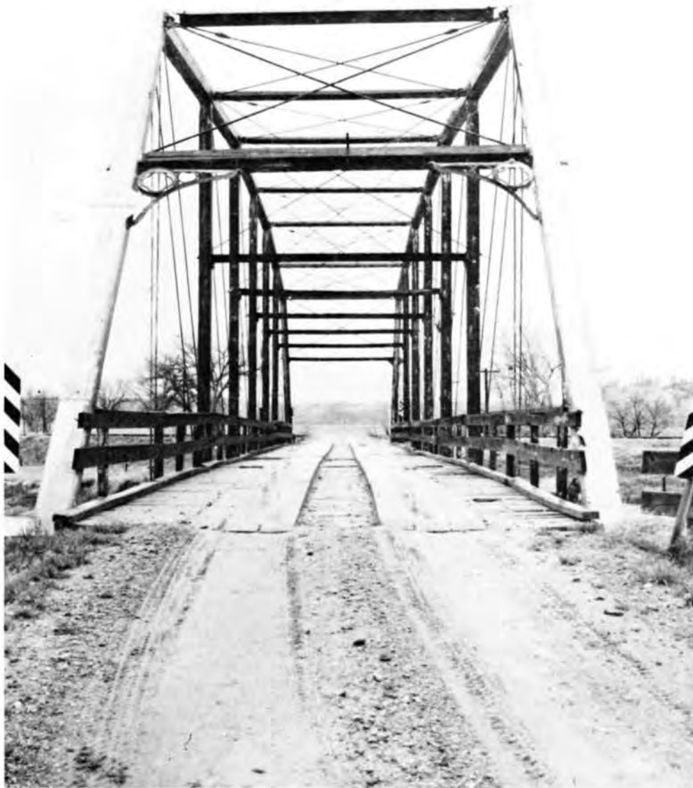
The Brockway Ford Bridge (Description 54) is the oldest remaining wooden truss in Montana. (Photograph Jet Lowe)
