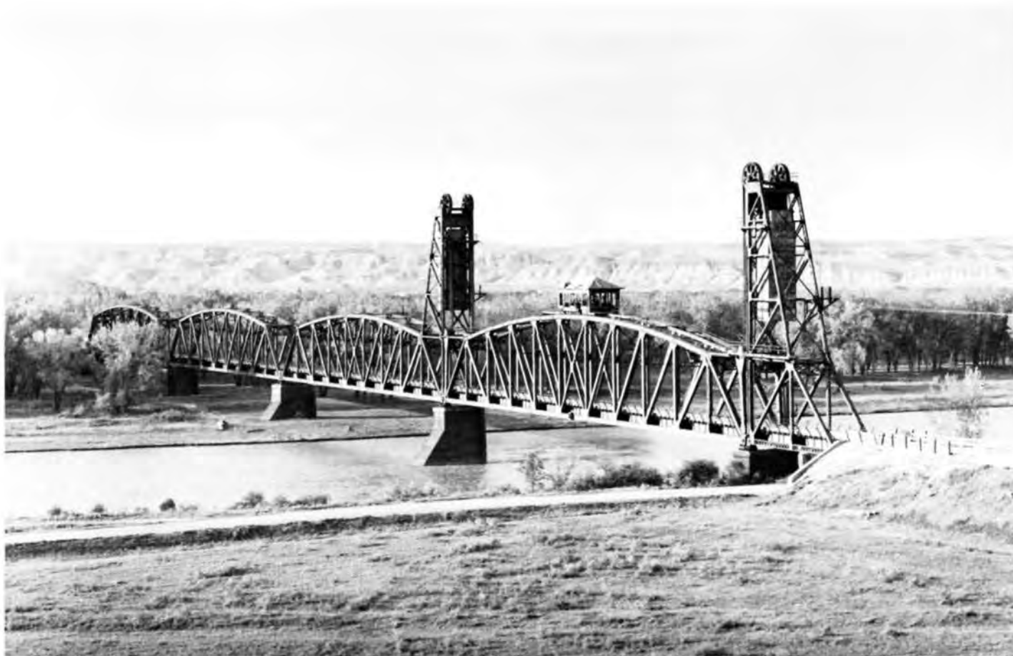
The Snowden Bridge (Description 65) was built in 1913 over the Missouri River. (Photograph Jet Lowe).
