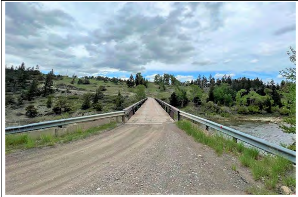
Figure 3. Sun River Bridge (24TT199), overview; view northeast. Photo by Jeannie Larmon, 5/24/2023.
