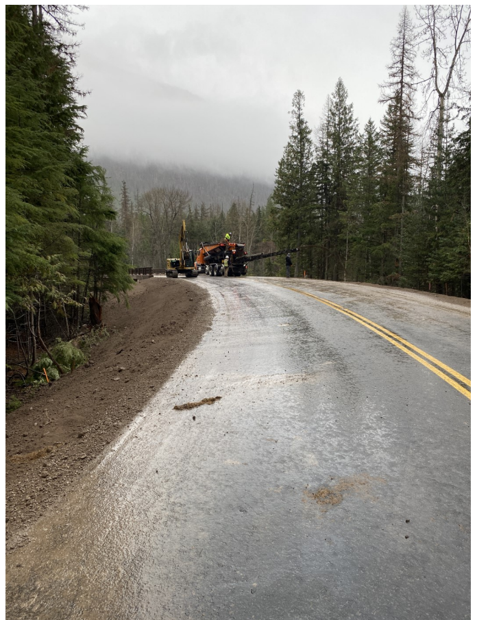
Upper McDonald Creek Rd topsoil placement
