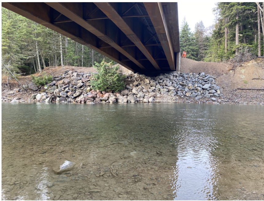
Abutment 2 rip rap after removal of old bridge
