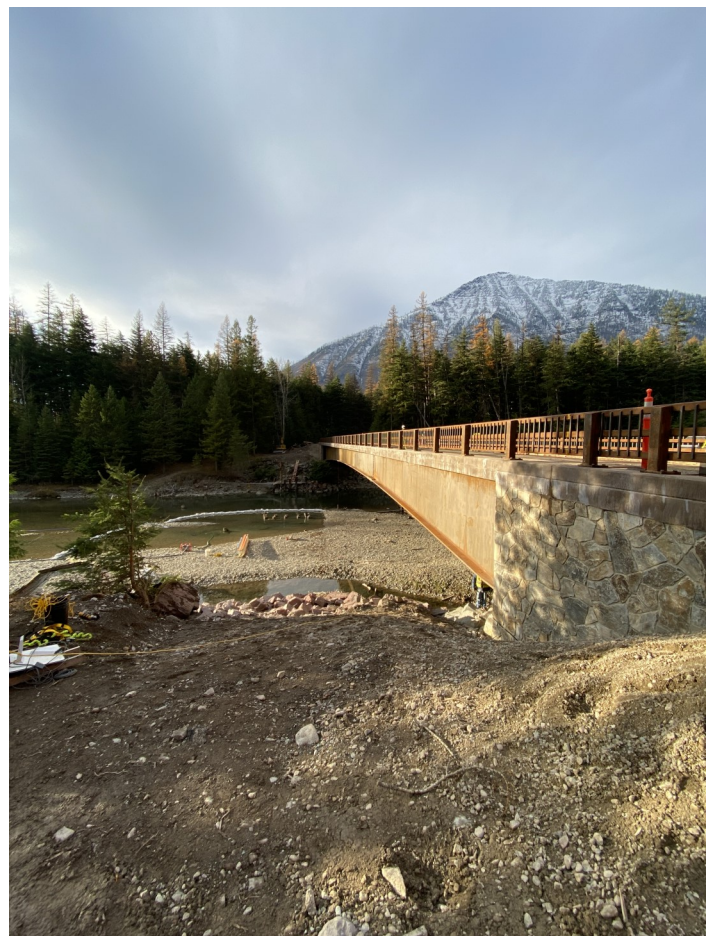
Alignment from old bridge during demo operations
