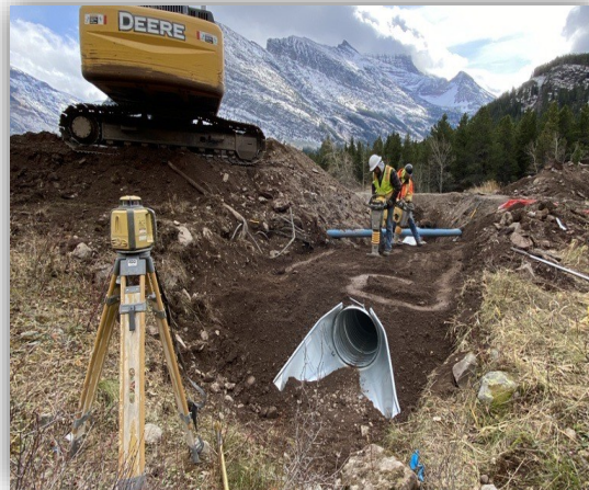
Culvert Installation
