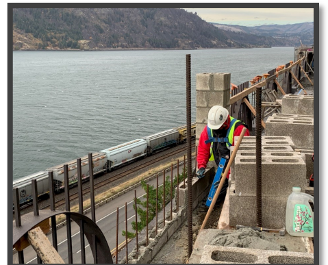
Installing the CMU Block Wall On the West Bench
