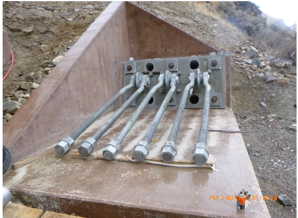
Installation of the Open Bridge Socket take-ups on EAB 2B
