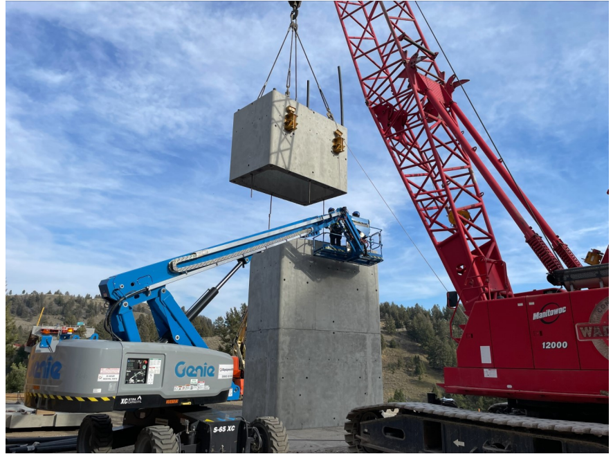
Erection Of Pier 1
