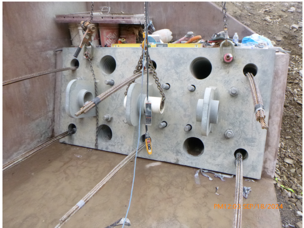
Test Fitting of EAB 2A Base Plate
