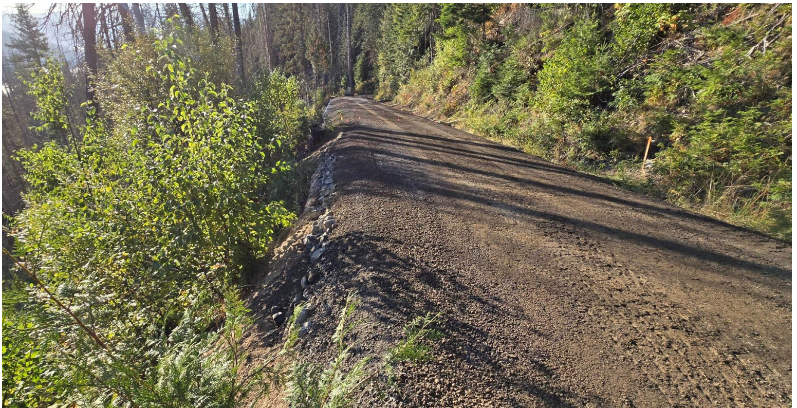
Completed roadway and shoulder improvements FSR 470 M.P. 2.52
