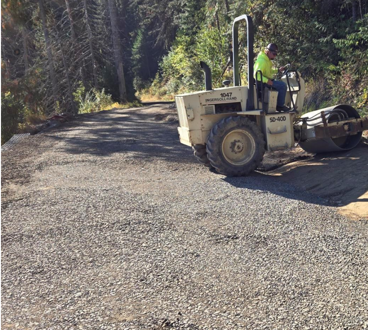
Sub grade and ditch line construction FSR 470 M.P. 2.52 Source: FHWA
