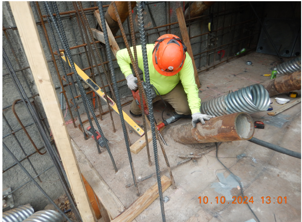
Reinforcing steel at Abutment 1 anchor block
