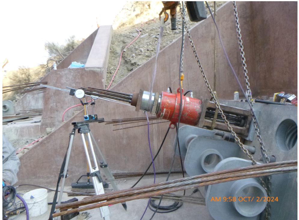
Proof Testing of EAB 2B #2 Ground Anchor
