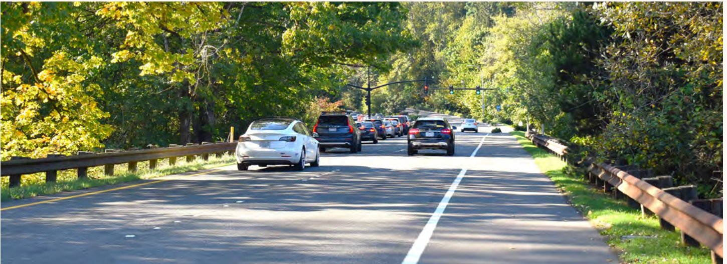
Figure 26: Lake Hills Connector—a two lane (by direction) roadway is physically separated from opposing traffic—runs east-west through Bellevue and provides an example of a Suburban 40 mph arterial.
