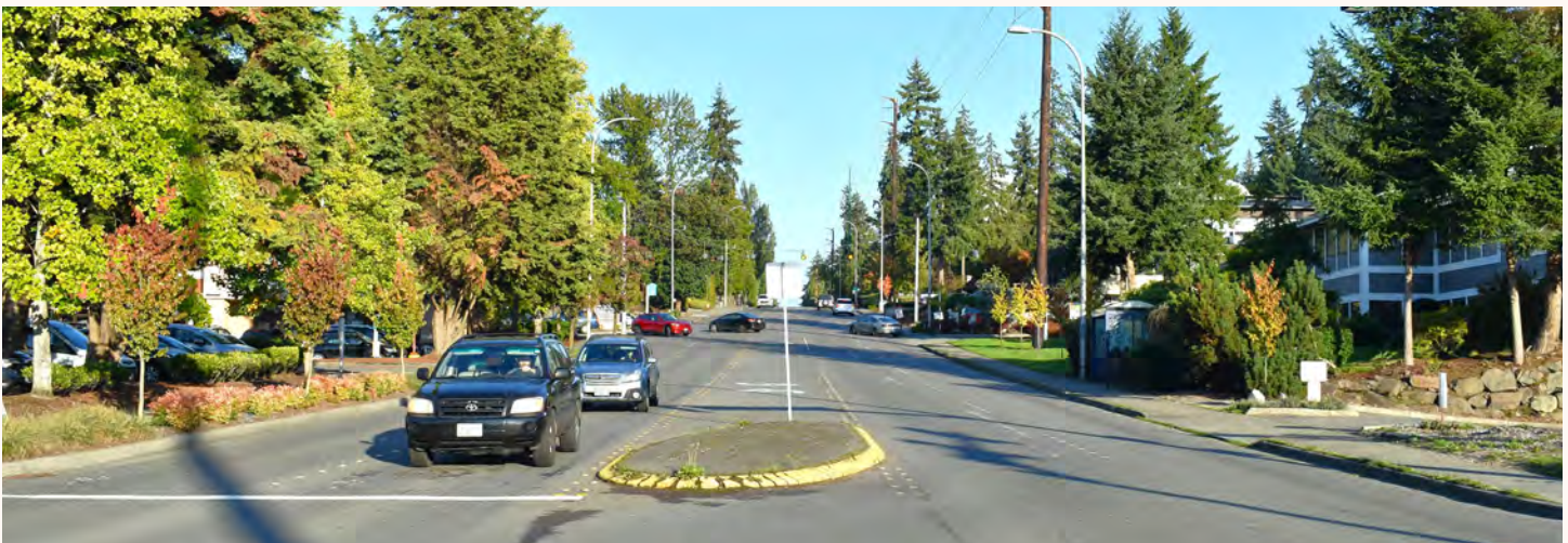
Figure 16: NE Eighth Street along the Crossroads commercial area provides an example of an Urban 30 mph arterial.
