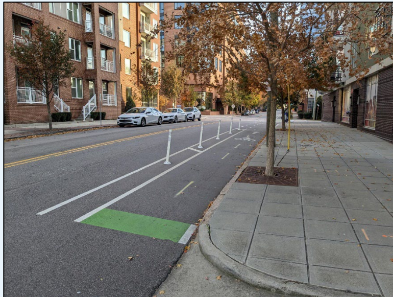
Figure 22. Photo. Illustration of a separated bicycle lane (i.e., horizontal and vertical separation).
