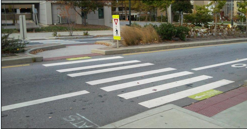
Figure 68. Photo. Illustration of a marked crosswalk with refuge island and supplemental devices.
