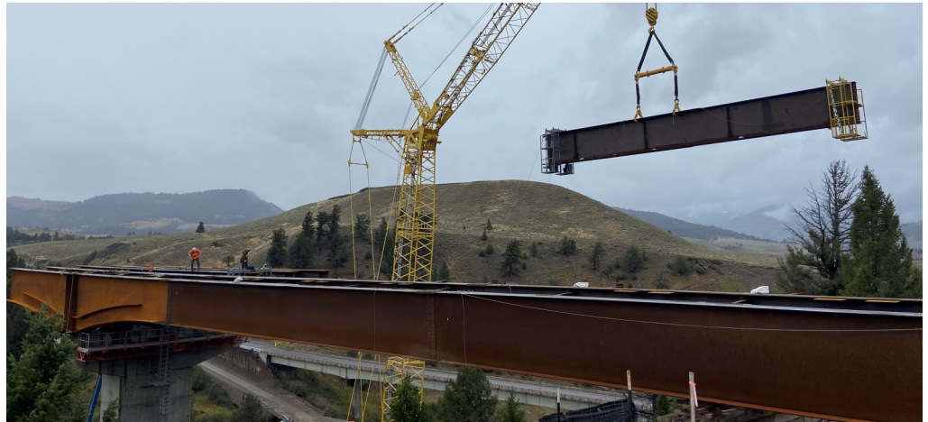
Girder Erection Span from Pier 3 to Abutment 2
