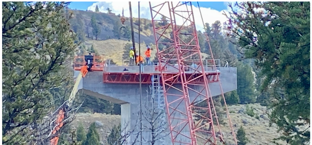
Installing Strands on Pier 2 for Future Post Tensioning
