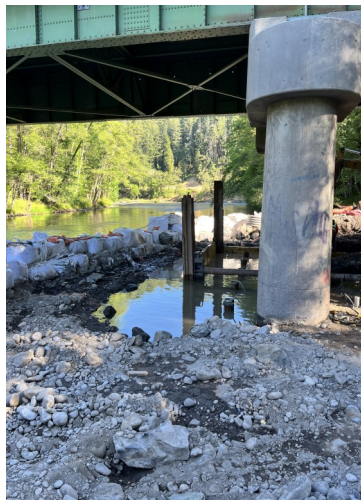
Shoring at Pier 4—Barnard
