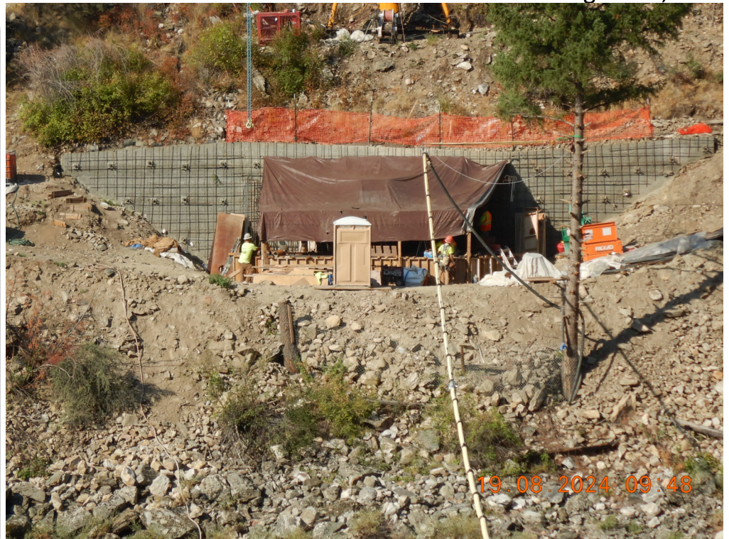
Abutment 1 viewed from the north side of the River
